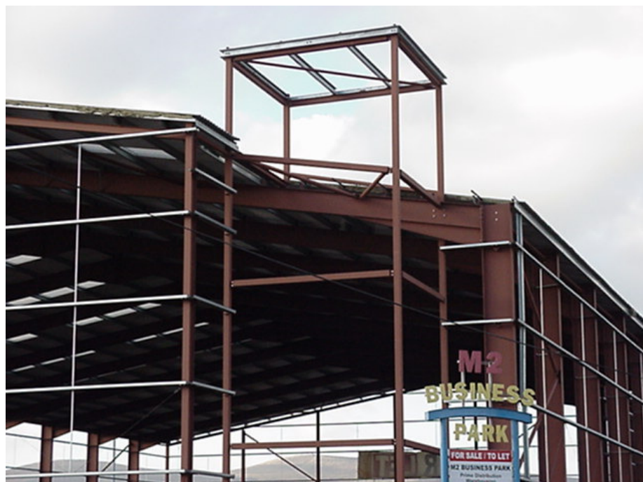
Figure 13 – Panel Support Frame
